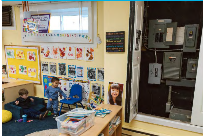
Before - Out-Of-Compliance Electrical Panels
