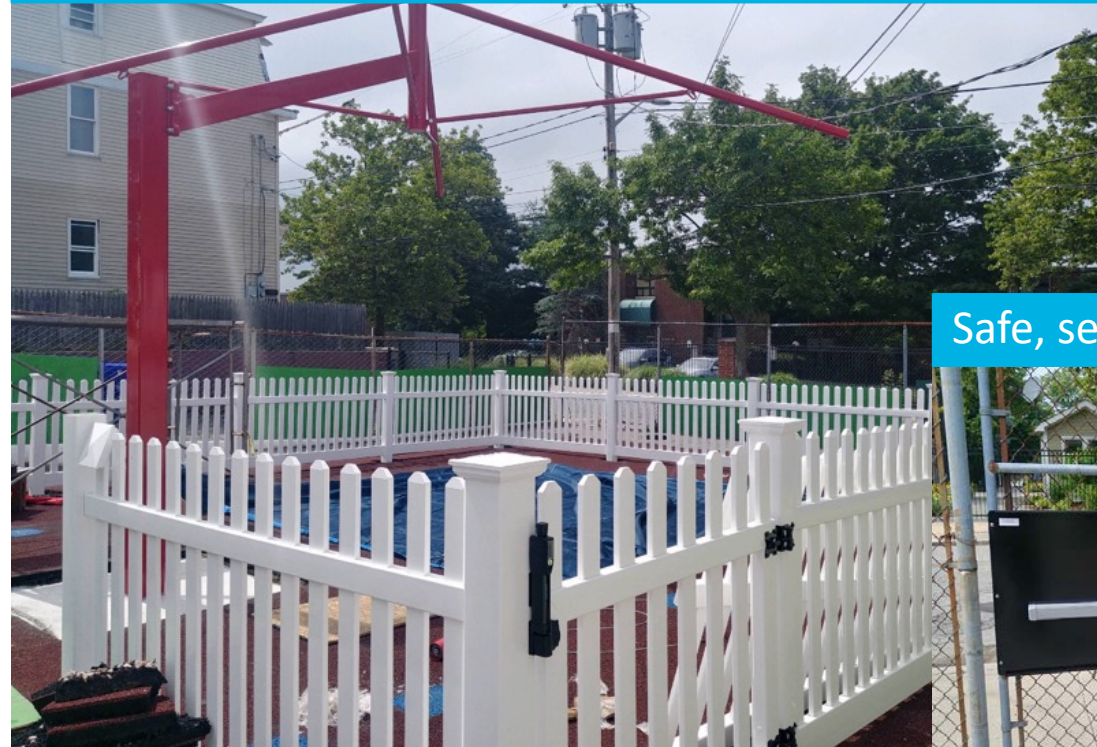
New fencing and shade for play space
