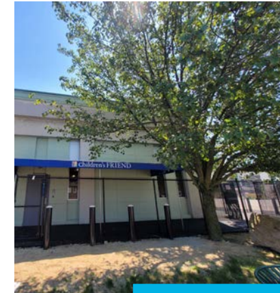
New Outside Fencing
