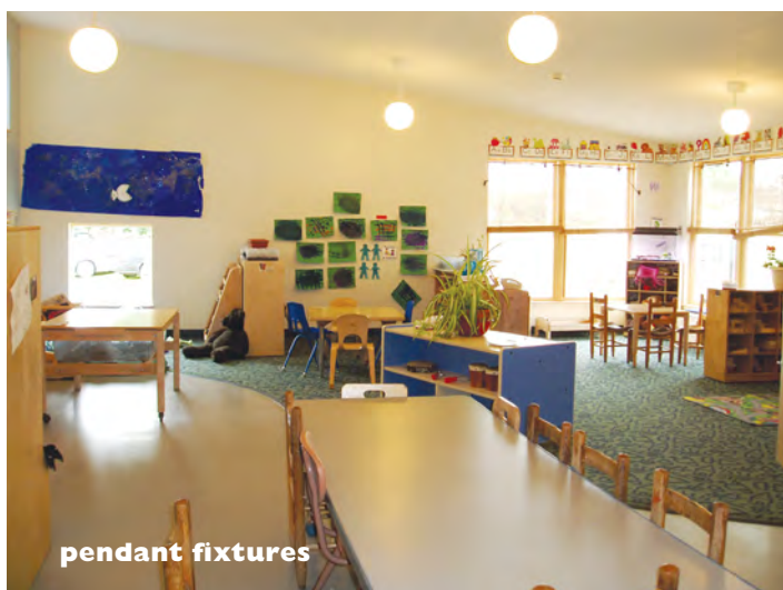
ABOVE: These pendant light fixtures suspended from the ceiling use incandescent bulbs to produce soft, multidirectional ambient light. These unshaded lights should not be used with high-watt bulbs, because they will create glare unless the amount of light is carefully controlled with a dimmer switch.
